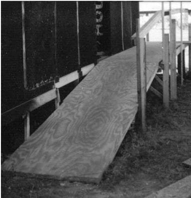
One side and all rear exit doors bring the customers to the front of the building via this ramp. Note the wood is not painted. It is treated with several coats of water seal. The end of the ramp is smoothed out with dirt and gravel. All exits must be ramped. A dark attraction may not have any steps inside or out.
