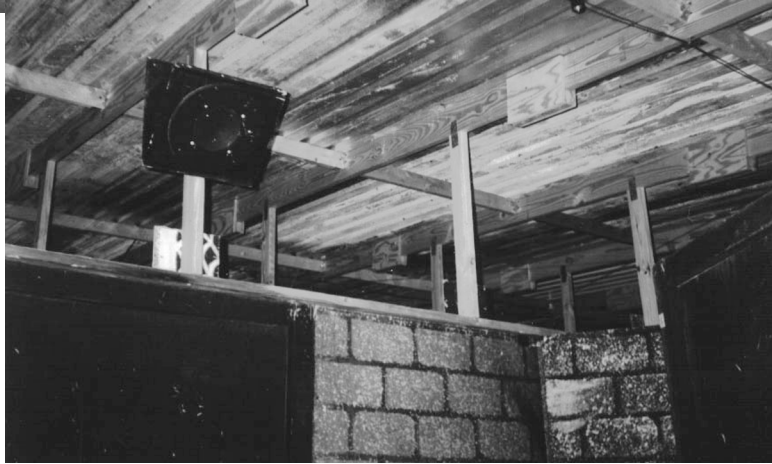
View looking up at roof. Note roof support system, joist connector and 70 volt speaker.
